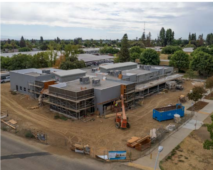
Construction of the Center for Early Childhood and Education.
