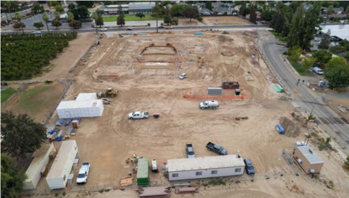
Construction of the Center for Fine and Performing Arts.
