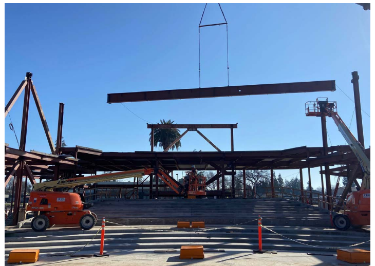
Beams (plate girders) going up on the CFPA.
