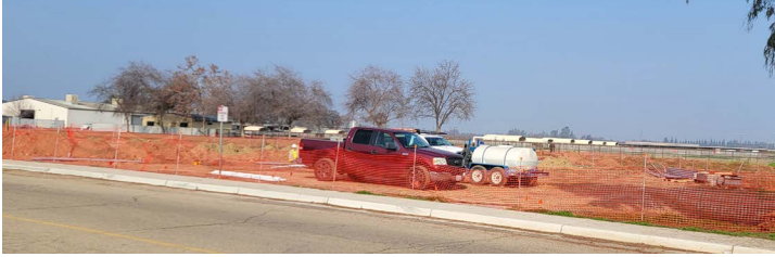
PG&E crews have started their work at the site.
