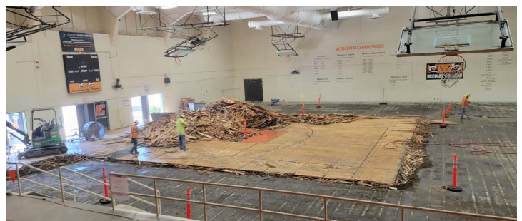
Demolition of the old gym floor started in early March.
